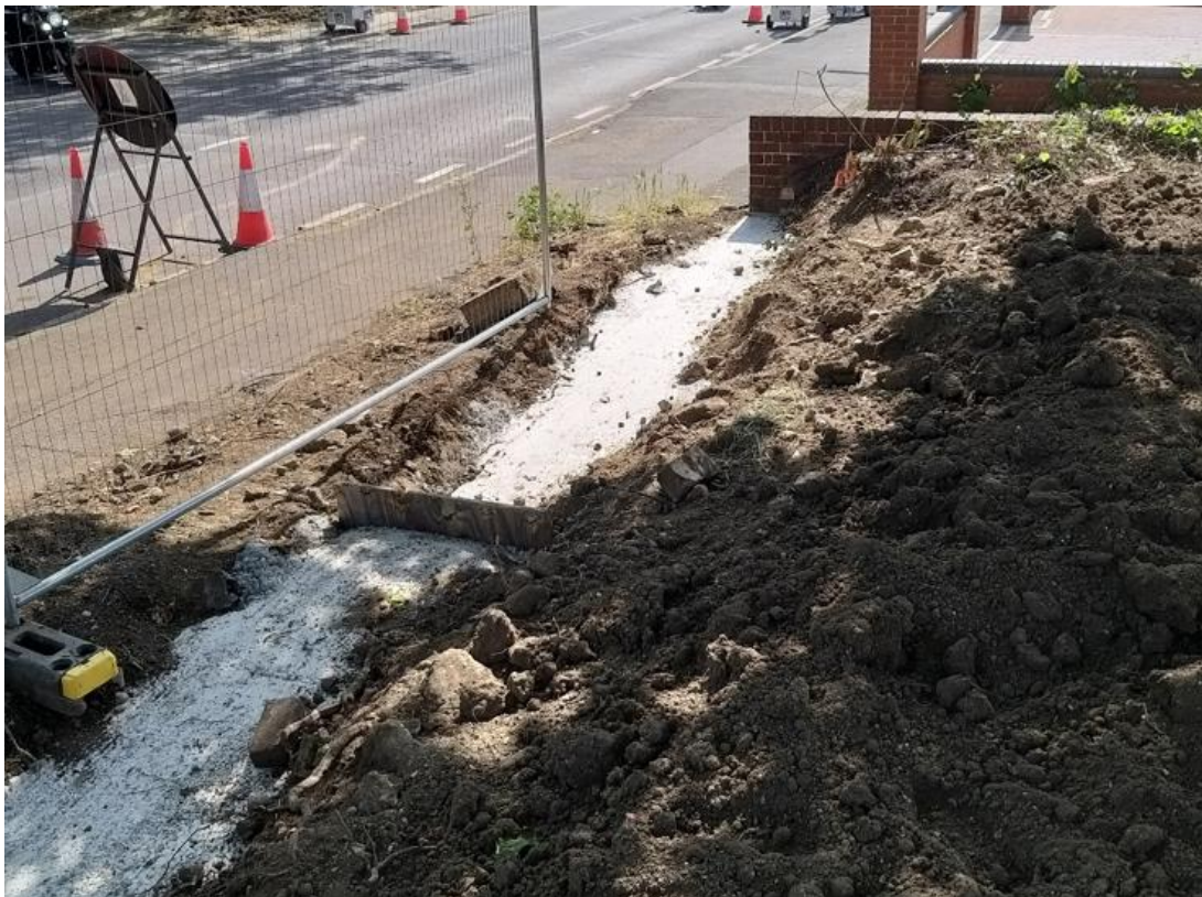
New foundataions on boundary with Manor Road (T1 out of shot to the right)
